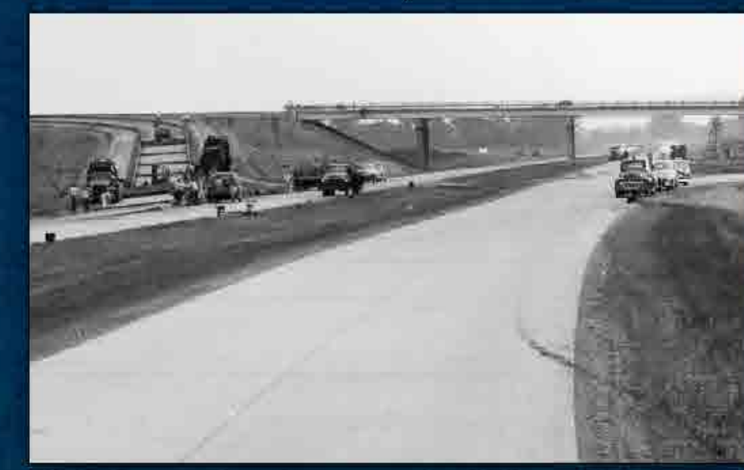
1954 Construction of access road on US Route 23
