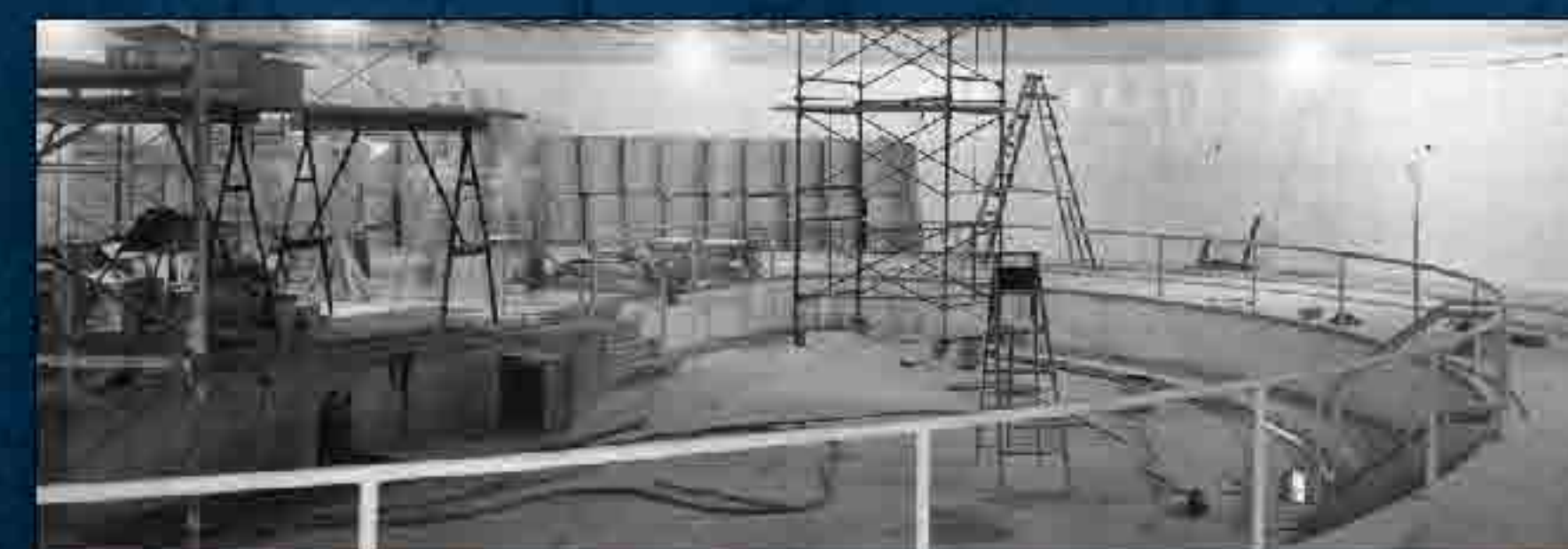
1954 Interior view of X-300 Plant Control Facility
