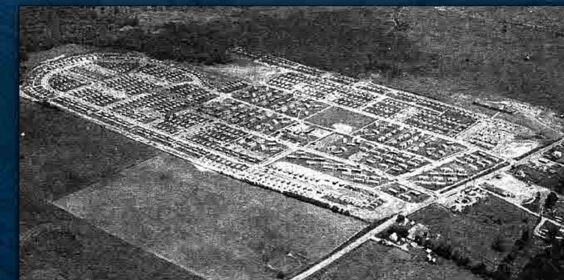
1954 Worker camp aerial view
