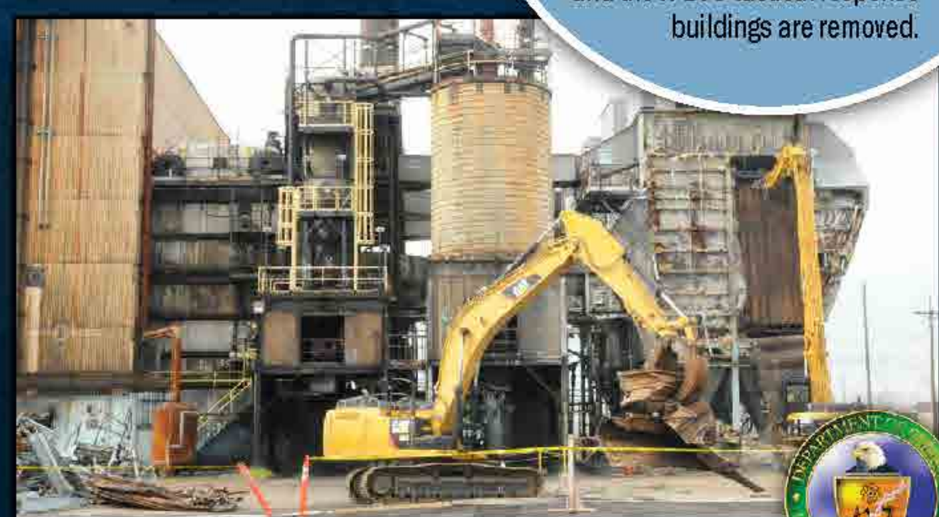
2016 Demolition of the X-690 Steam Plant
