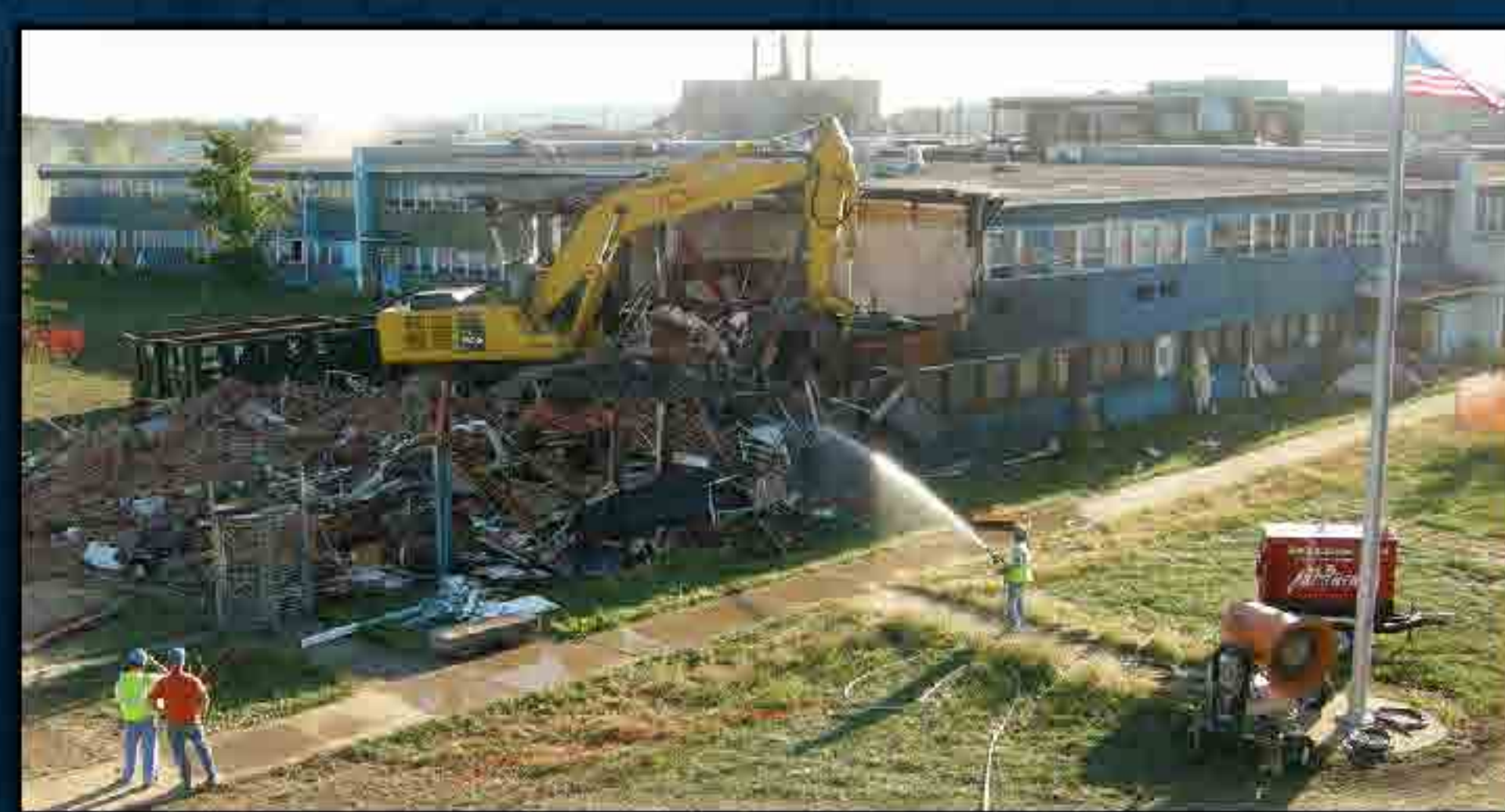
2012 Demolition of X-100 Administrative Building
