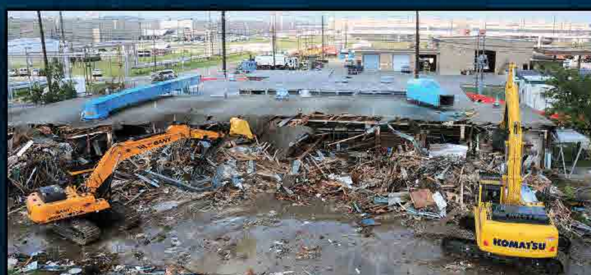
2013 Demolition of the X-102 Cafeteria
