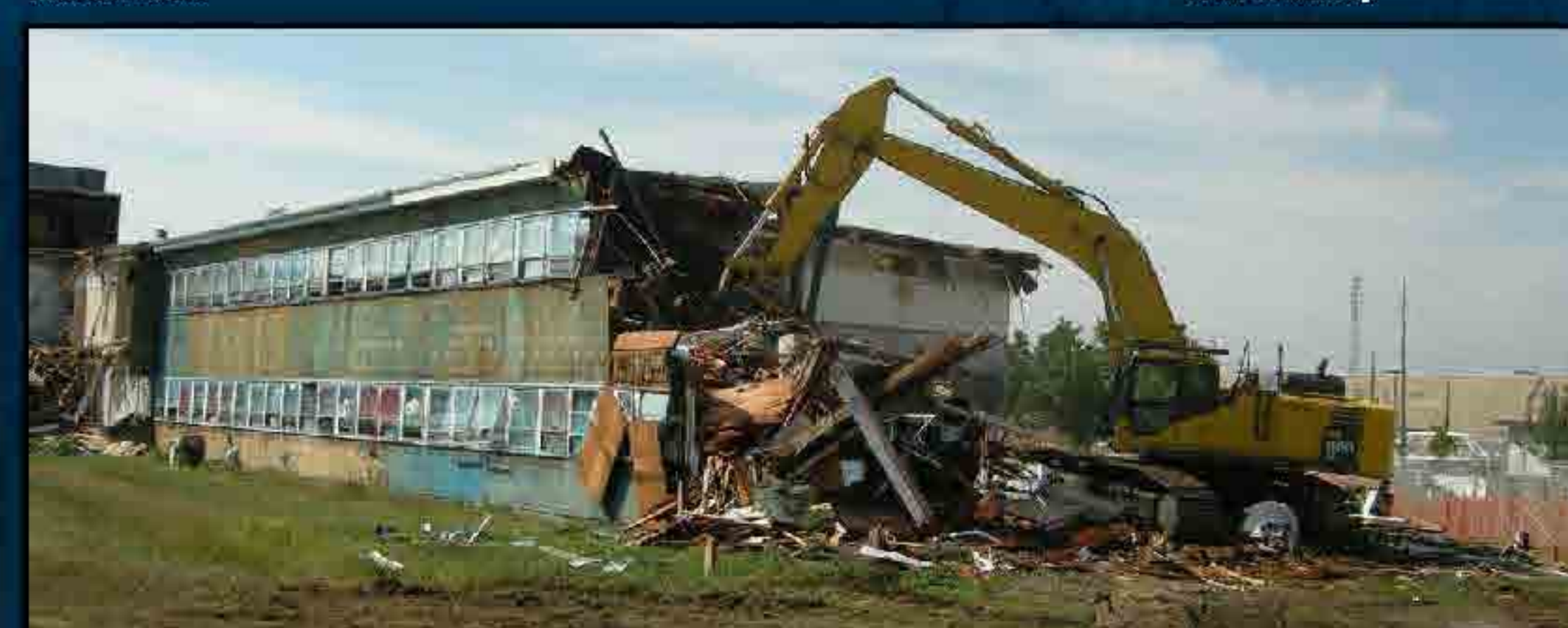
2012 Demolition of the X-100 Administration Building
