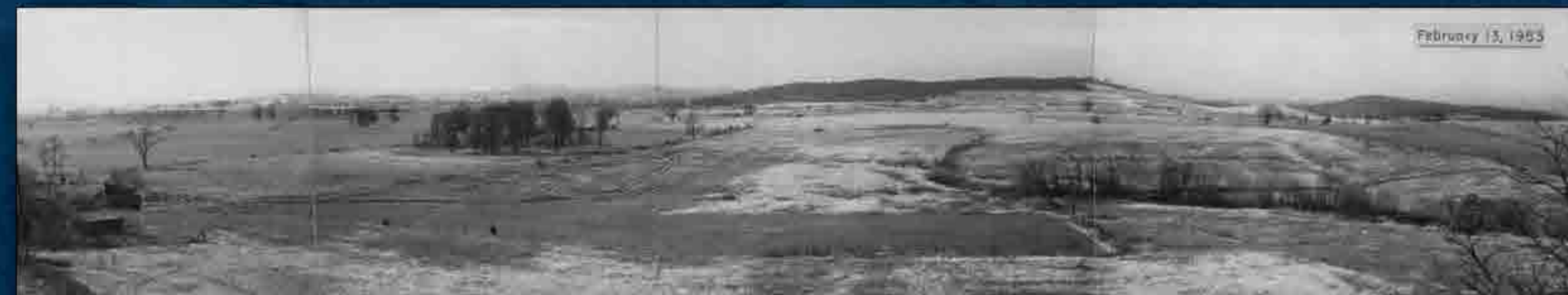
February 13, 1953 The site before construction begins
