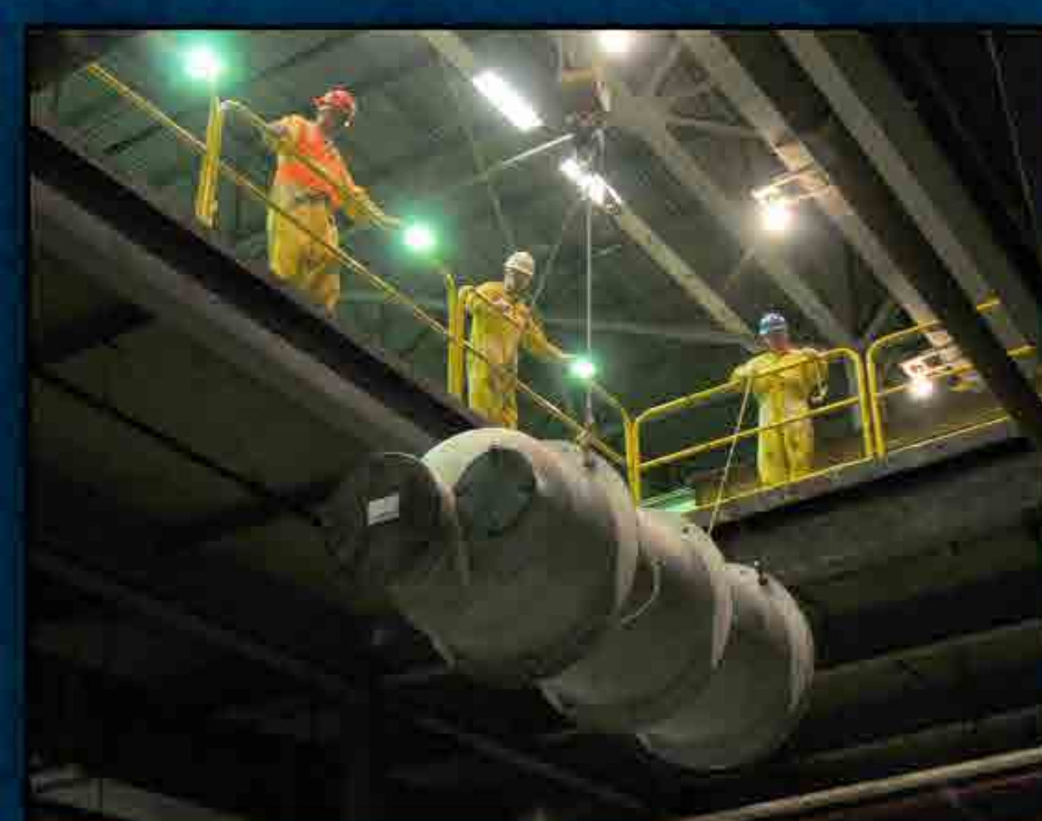
2012 7,000 components removed in the X-326 as part of the deactivation
