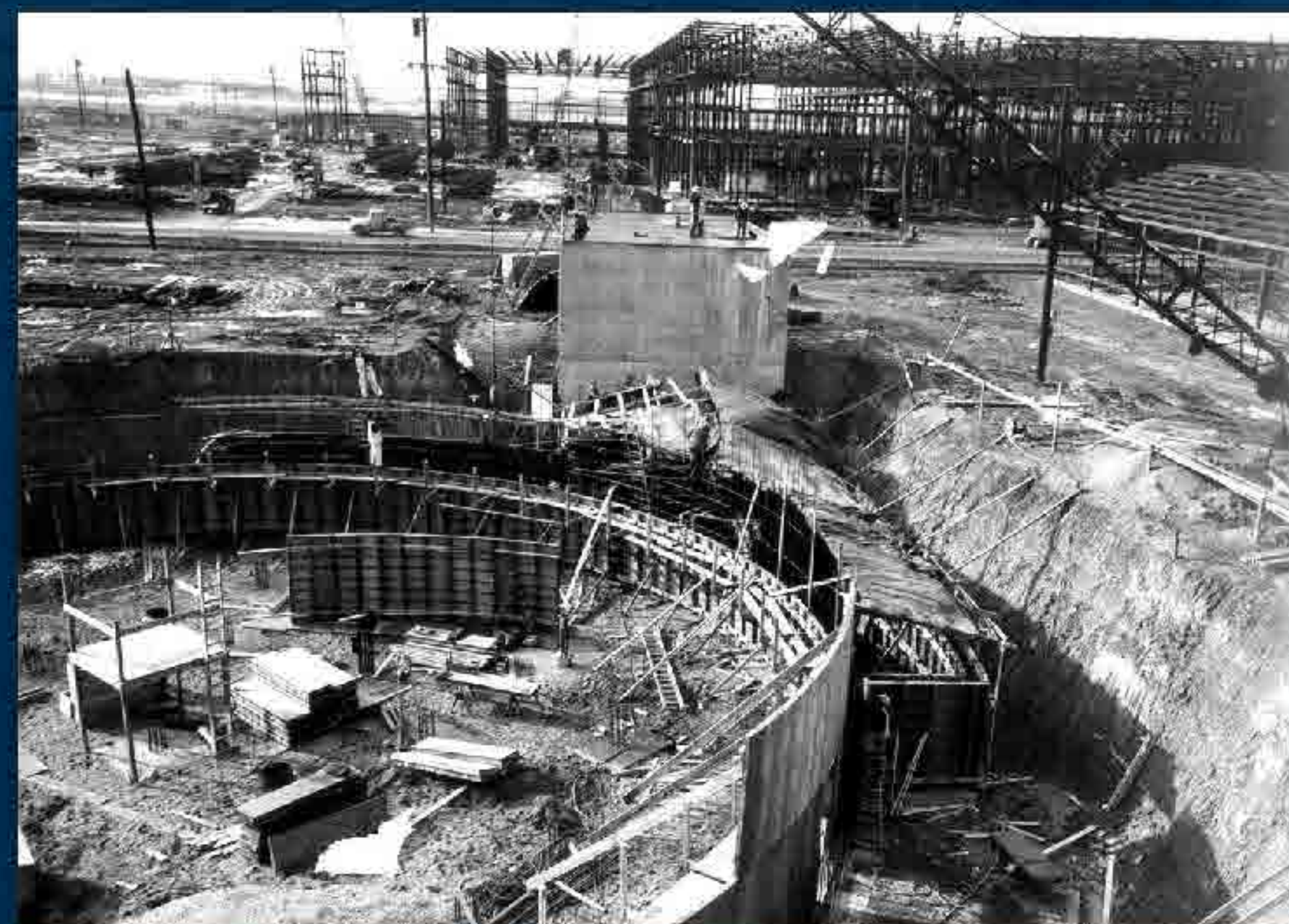
1953 Plant Control Facility X-300 construction
